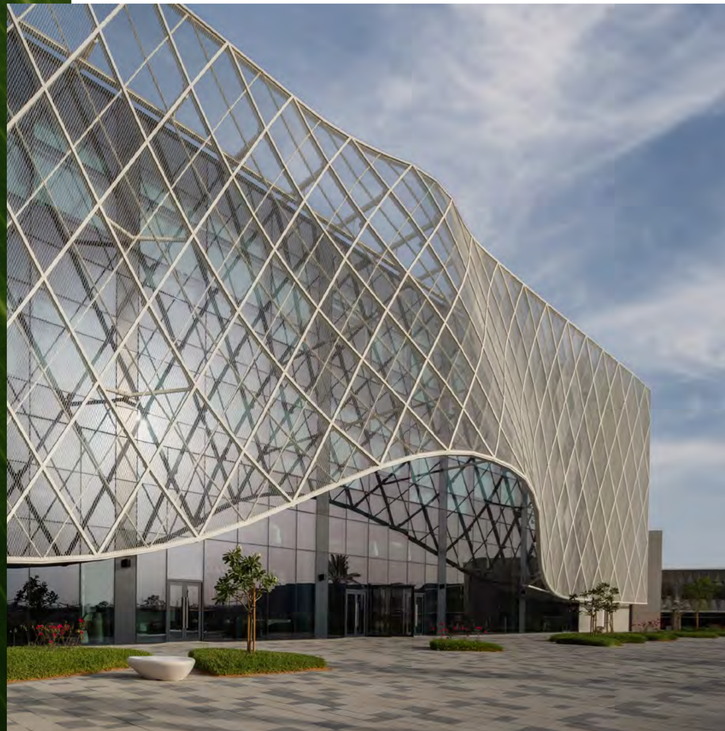
Aldar HQ, Abu Dhabi
